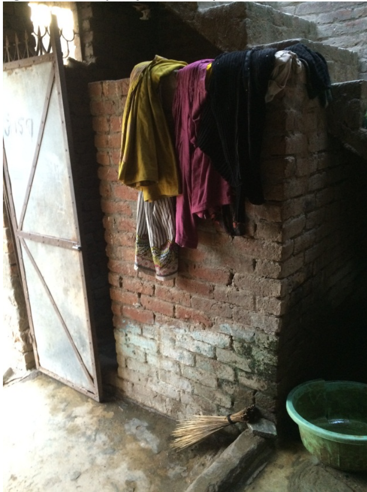
Figure 2b: Example of an Unacceptable House
